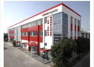
New Suzhou facility
