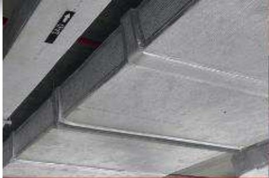
Duct Insulation
