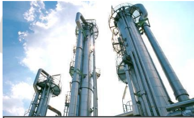
[Oberhausen, Germany] Oberhausen Plant TOPAS Advanced Polymers GmbH
