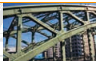
Measurement of corrosion protection coatings in harsh environments
