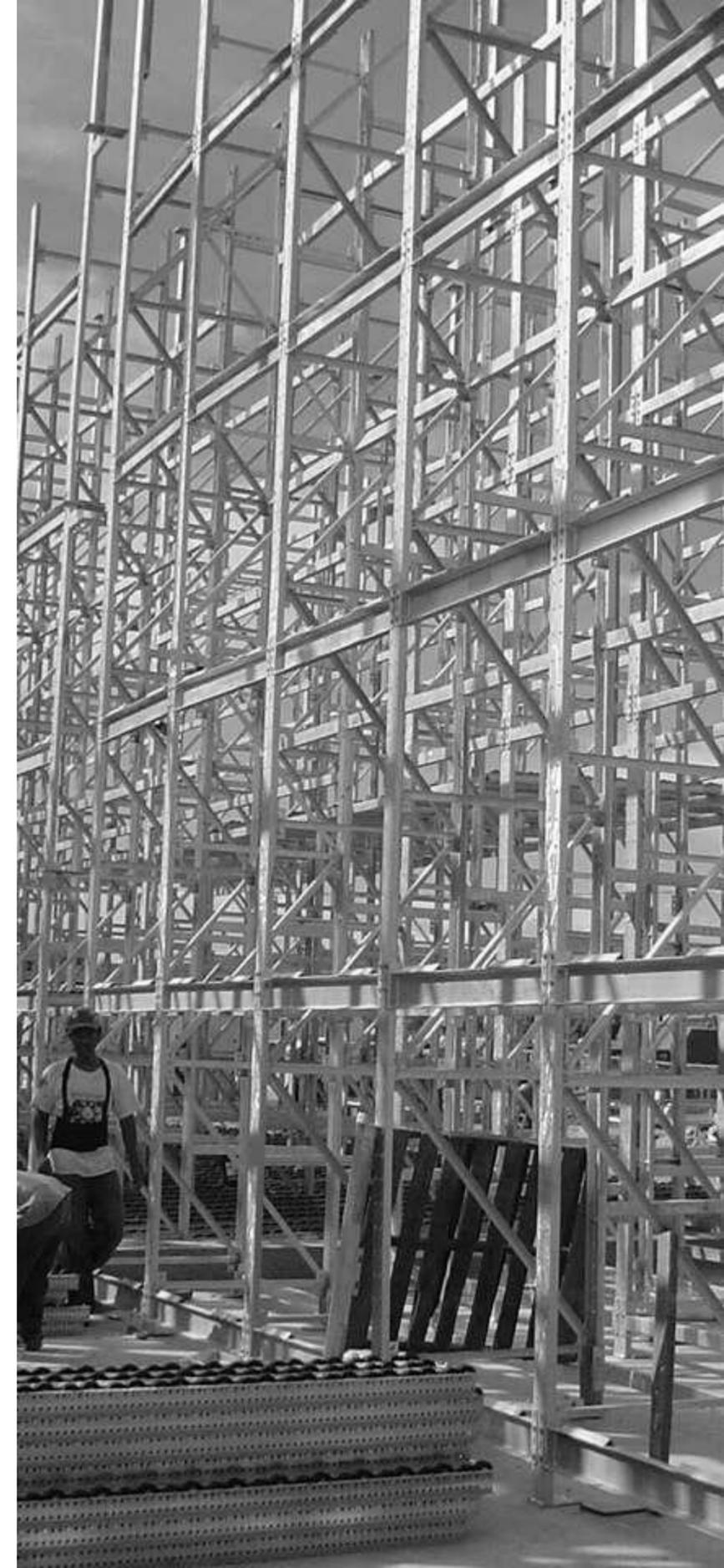
A self-supporting system is a system that integrates the shelf as a supporting structure of the whole construction.
