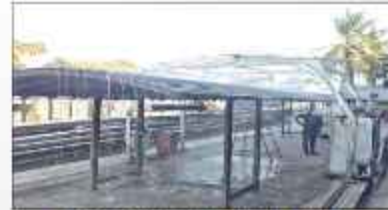
ROOF SHOWER LEAK TEST
